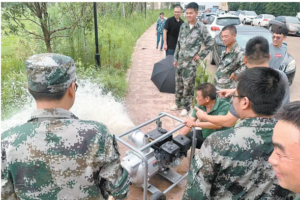
筑牢防汛堤坝
